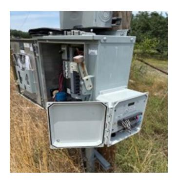
Additionally, each unit features a backup battery, ensuring continued operation and communication even if power to the system is lost. This guarantees alert functionality during outages or potential theft events.
